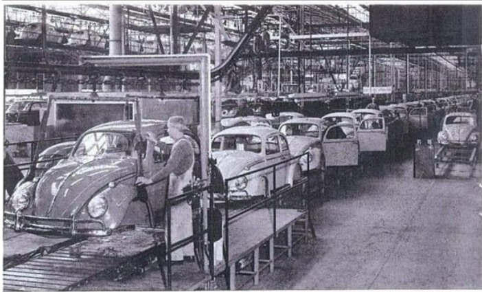
The main VW 1200 production line at the Clayton, Victoria, plant of Volkswagen Australasia Ltd. Plant capacity of VW 1200 sedans is more than 100 vehicles a shift.
