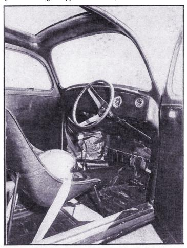
Interior of the car is very Spartan. The skylight is filled in with plastic.
