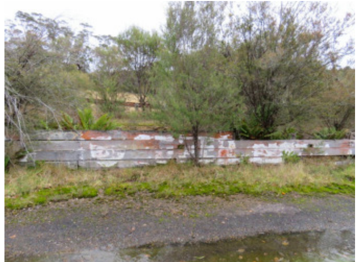
Very faded BP Super sign on the KLG Straight Fence
