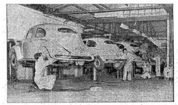
General view of the workshop area showing part of the battery of hydraulic hoists which speed up the servicing of vehicles. As a general rule all vehicles are hoisted for ease of working. Such modern works shop conditions permit the mechanic to have the vehicle at a suitable height for the particular job, and ensure speedy and efficient work.
