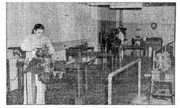
The ongine unit reconditioning section at Greg Cusack's Service Station contains a wide range of jigs and special machine shop equipment specially designed for Voltswagen maintenance. In the foreground Charlie Beswick, the workshop foreman, is reassembling a <u>YW</u> engine which is conveniently held in the special roll-over jig.
