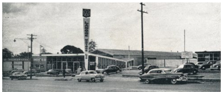
General view of Lanock Motors Ltd., Five Dock Branch.
