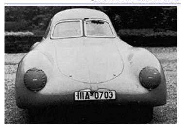
The car weighed 545 kg, 200 kg less than the normal KdF sedan. It reached a maximum speed of 145 km/h, and thanks to excellent testing results, appeared to be absolutely ready for the forthcoming race.
